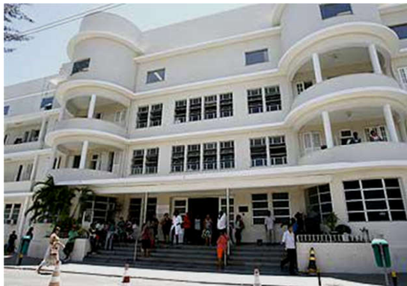
Figura 1 – Hospital Aristides Maltez
